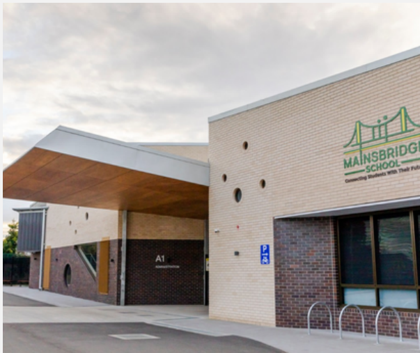
Mainsbridge SSP - Warwick Farm
